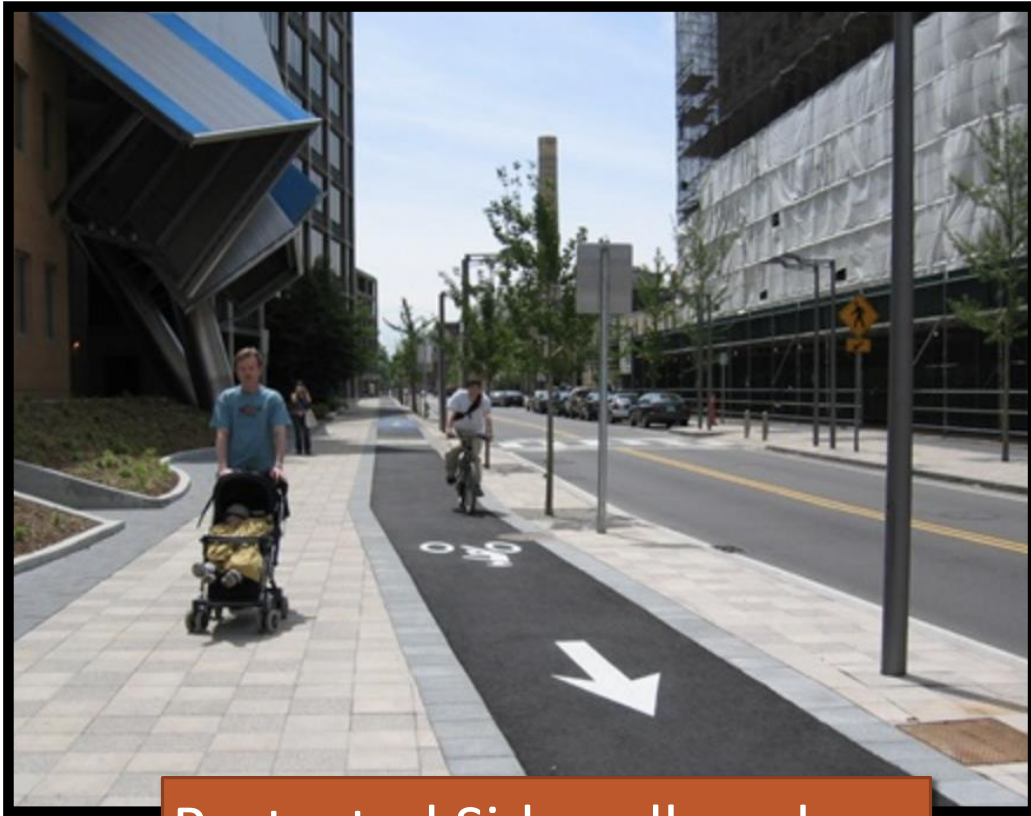
Protected Sidewalk and Bike Lane in Cambridge
